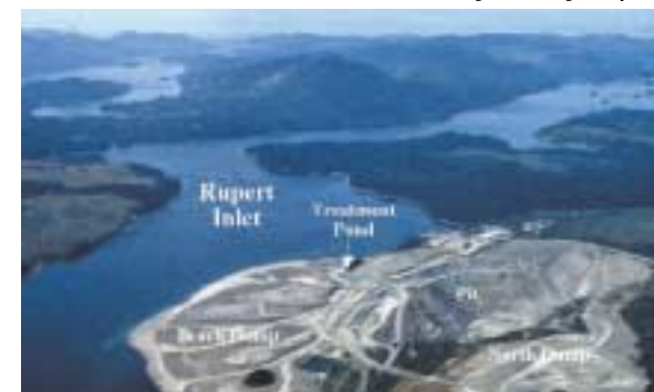
Aerial photograph of Island Copper during operation.
